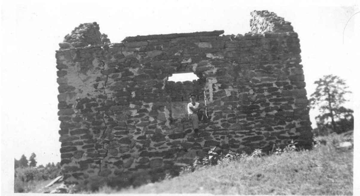
Teachout barn foundation remains – Local Historian Forest Porter Photo taken in the 1960's timeframe
